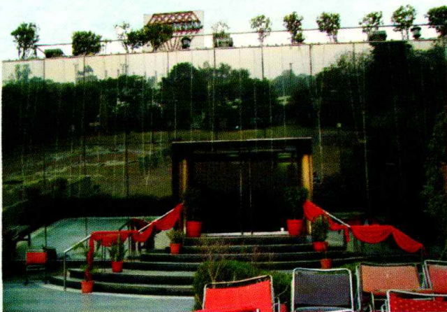
Crystal Banquet Hall, Pragati Maidan, Delhi Client : R.K. Gupta & Associates, Delhi Architect : Narayan Murti, Vasantkunj, Delhi Project Value : (Aprx.) Rs. 19,50,000.00
