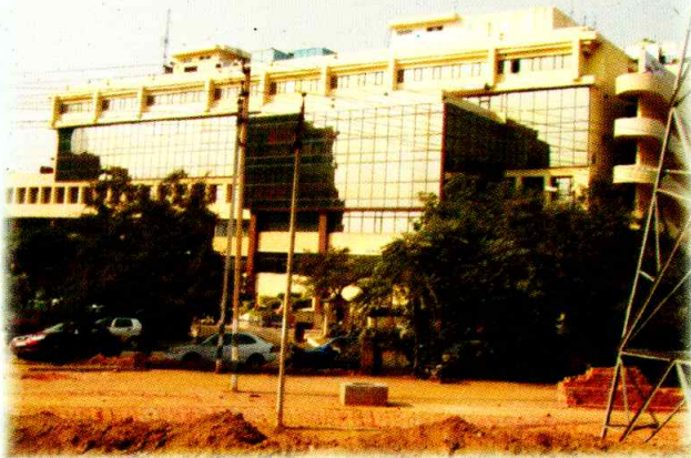
N.K. TOWER, N.K. Centre, Gurgaon Client : N.K. Towers (P) Ltd. Architect : Behal & Joshi Associates Project Value : (Aprx.) Rs. 78,00,000.00
