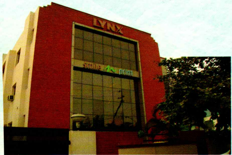
Lynx (Noida) Client : Lynx Printing Pvt. Ltd. Architect : Sharma & Associates, Noida Project Value : (Aprx.) Rs. 9,00,000.00
