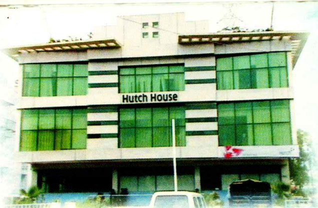
Hutch House, Shahnazaf Road, Lucknow Client : Ricco Structurals (P) Ltd. Architect : Abhigyan (Mr. Arun Kumar, Lucknow) Project Value : (Aprx.) Rs. 25,50,000.00
