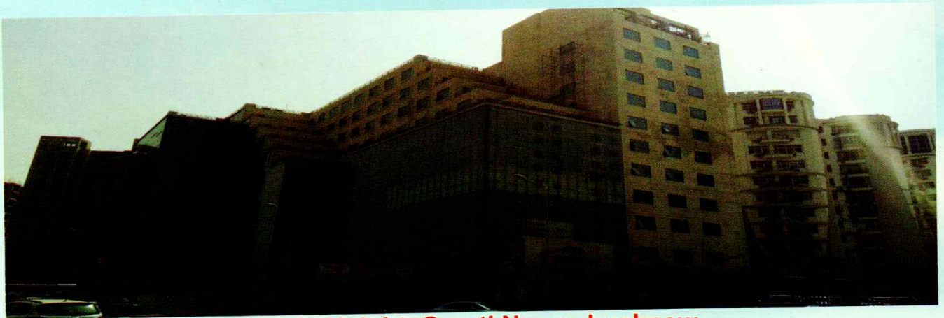
Cyber Height, Gomti Nagar, Lucknow Client : R.R. Civil Tech Pvt. Ltd. Architect : Design Group Project Value : (Aprx.) Rs. 4,54,00,000
