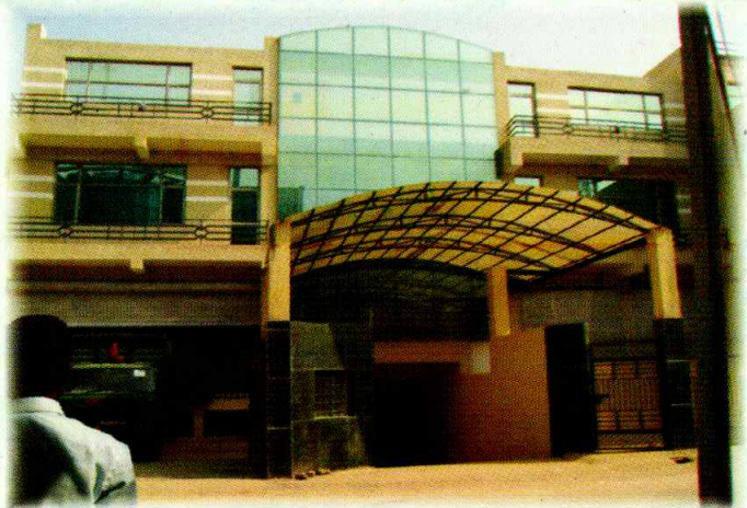
Packers Product, Kaspasheda Border, Delhi Client : Mr. Amit Choudhry Architect : Soni & Associates (M.S. Soni) Project Value : (Aprx.) Rs. 13,00,000.00
