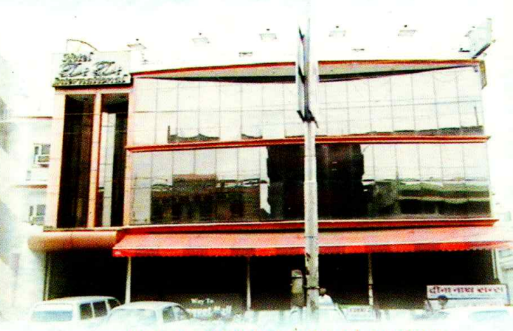
Hotel D.D. International, Lucknow Client : Deenanath & Sons, Lucknow Architect : Mr. R.K. Gupta, Lucknow Project Value : (Aprx.) Rs. 13,50,000.00
