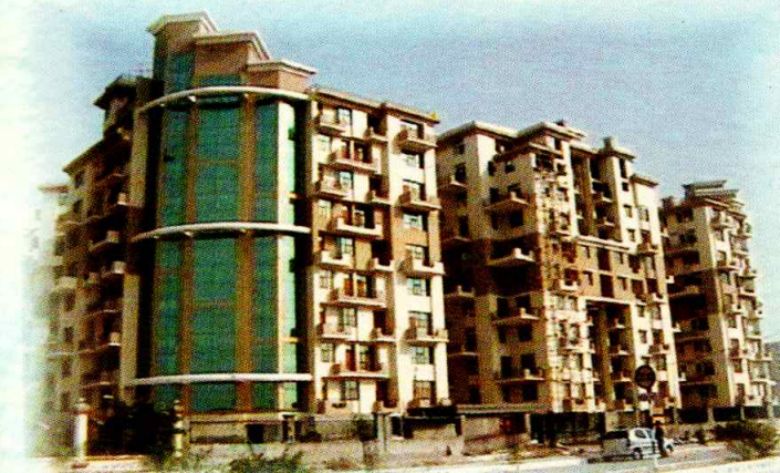
Best Buildwell Housing, Society, Dwarka Client : Best Buildwell (P) Ltd., Delhi Architect : Imagination, Mr. Vijay Goyal Project Value : (Aprx.) Rs. 85,00,000.00
