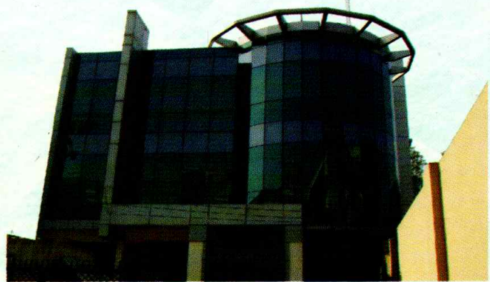
S.D.V. International, Delhi Client : Vikas Yadav (Kapasheda Border, Delhi) Architect : Mr. Narendra Gupta (Delhi) Project Value : (Aprx.) Rs. 17,00,000.00
